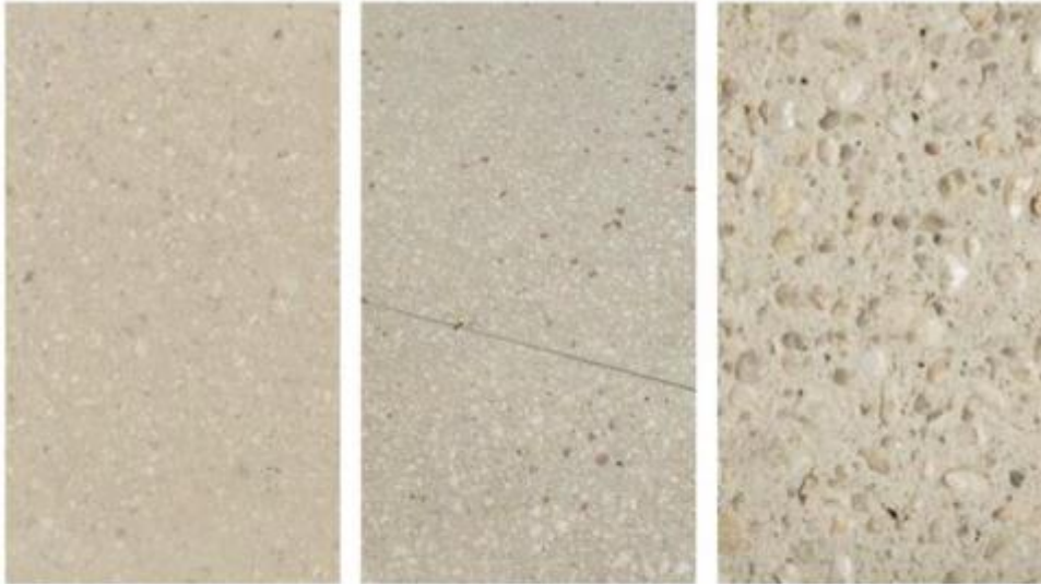
Figure 14: In-situ decorative surfacing etch and aggregate finishes ranging from the 0.5mm (left) to approx. 3mm (right)
