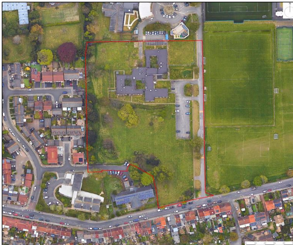
Figure 2 - Aerial view of site (prior to the demolition of the school building)
