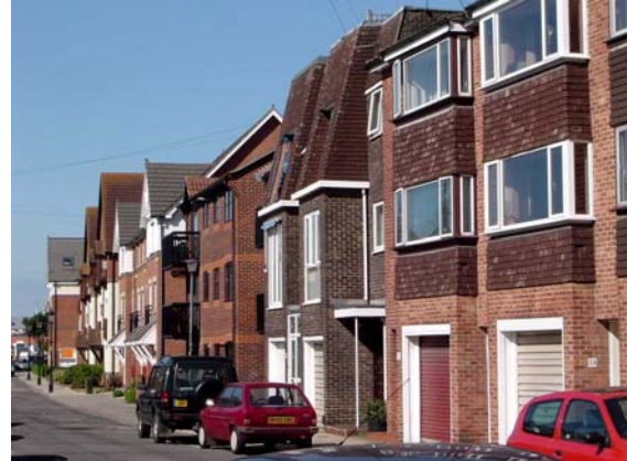
Most of the 1970s and 1980s developments on Warblington Street have allowed cars to dictate the design
