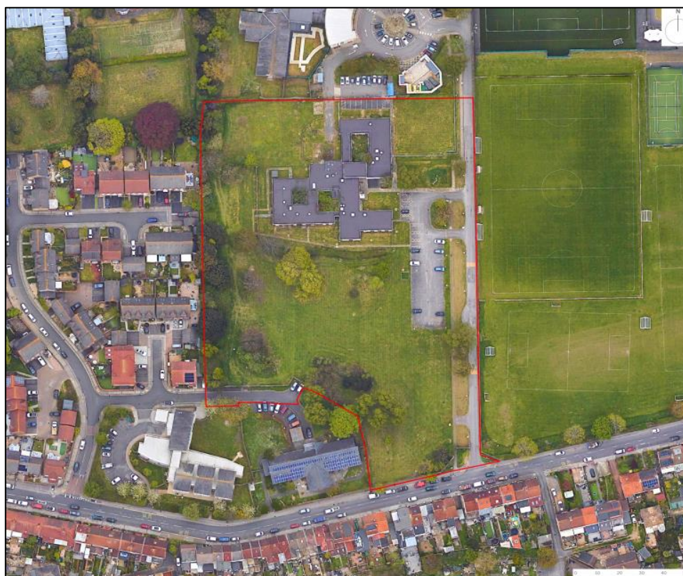
Figure 2 - Aerial view of site (prior to the demolition of the school building)
