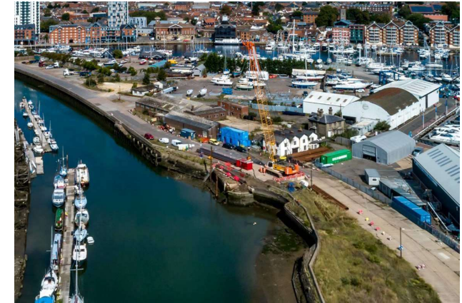
Quay Walls £16,300/m
