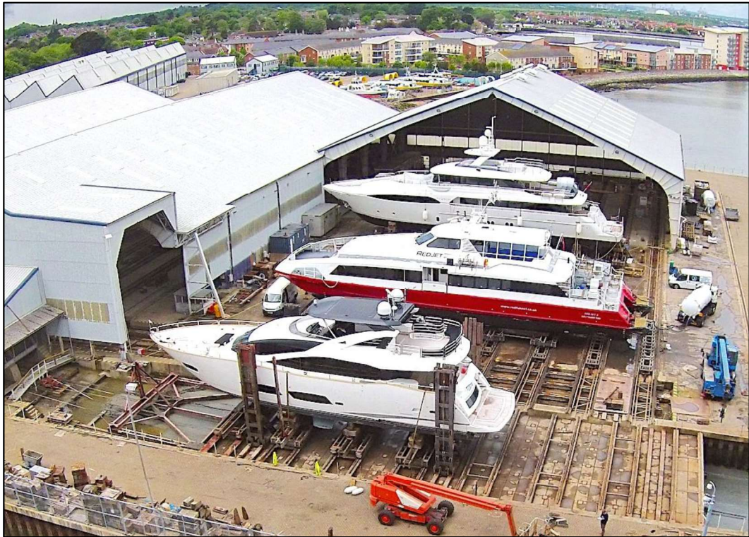
Figure 3.2 Solent Refit Boat Lifting & Storage Facility – Southampton Water
