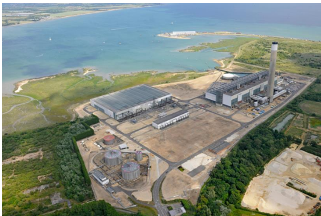
Figure 3-9 The Former Fawley Powerstation
