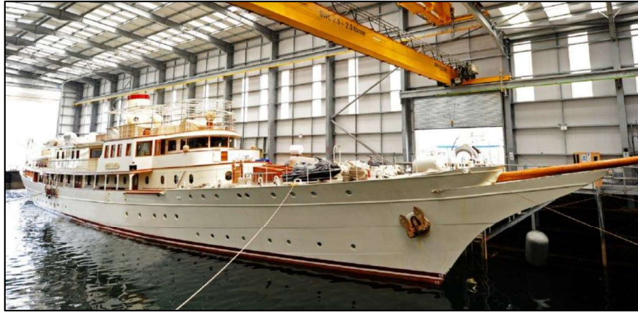
Figure 5.9 Pendennis Shipyard Dry Dock Falmouth
