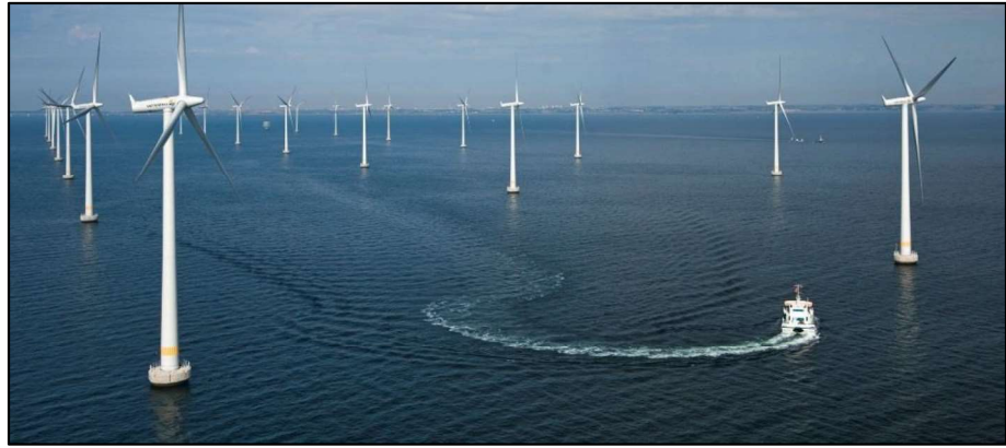
Figure 5.12: Typical Offshore Windfarm
