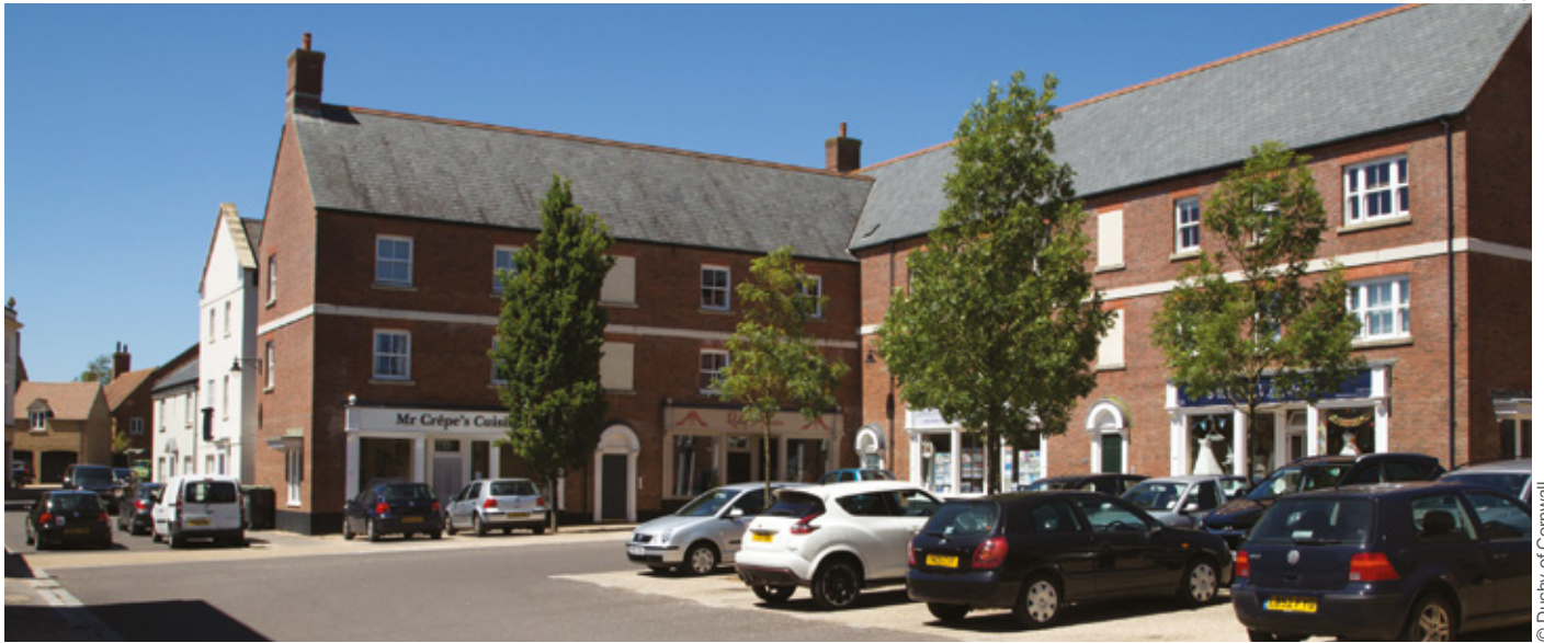
▼ Challowcombe Square, Poundbury
