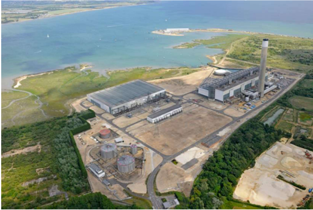
Figure 3-9 The Former Fawley Powerstation
